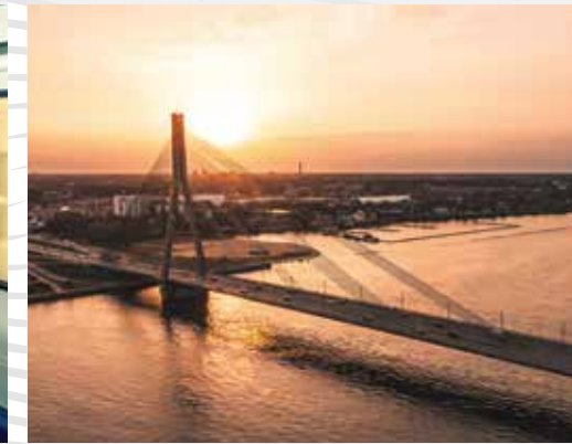
2 NEW BRIDGES OVER THANE CREEK SPEEDING UP MUMBAI-NASHIK TRAVEL
