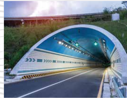
BORIVALI - THANE TUNNEL
